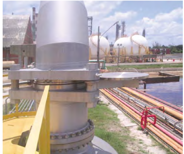
Cam-Set® DN 500 (20"), ASME 150# with spectacle plate support
