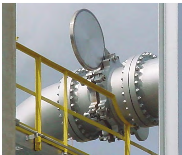
Stacey DN 850 (34") with counterweight
